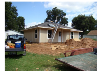
Jane's home nearing completion.
